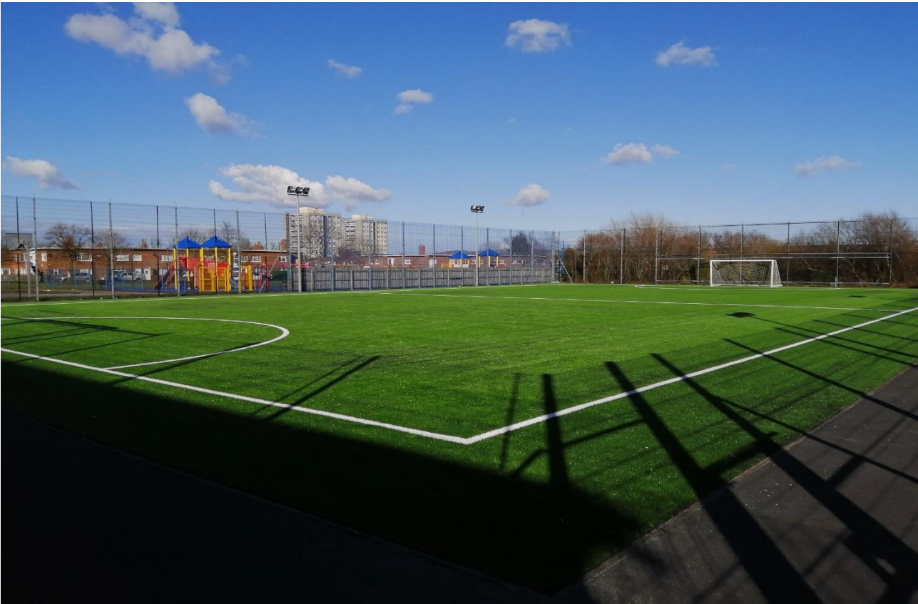
Cregagh & Shaftesbury 3G pitch carpet replacement
